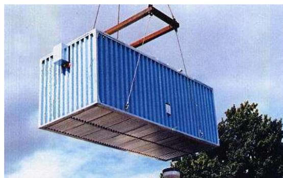
Figure 8 Portable heating and cooling bank
